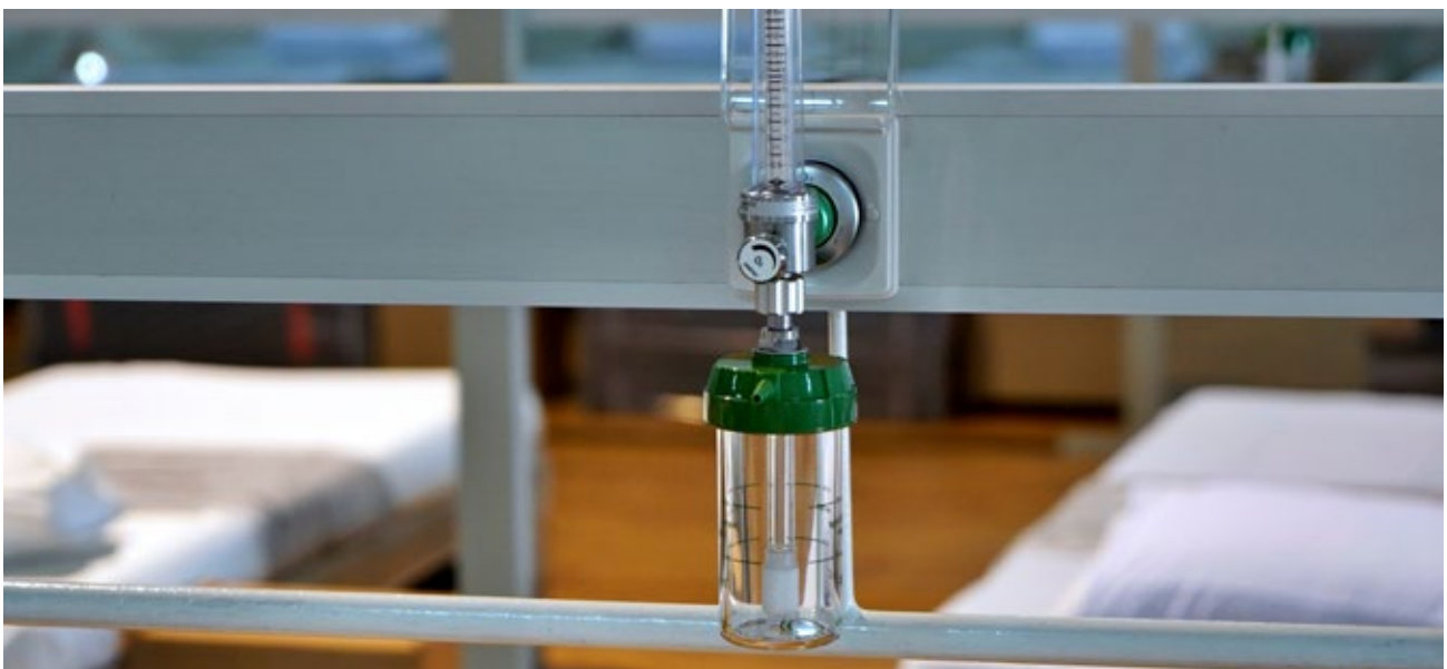
Saluran Oksigen Medis | Medical Oxygen Line
